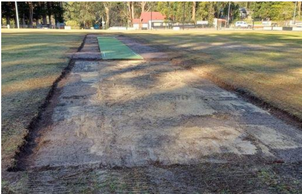
Artificial turf areas surrounding the wicket are being relayed
