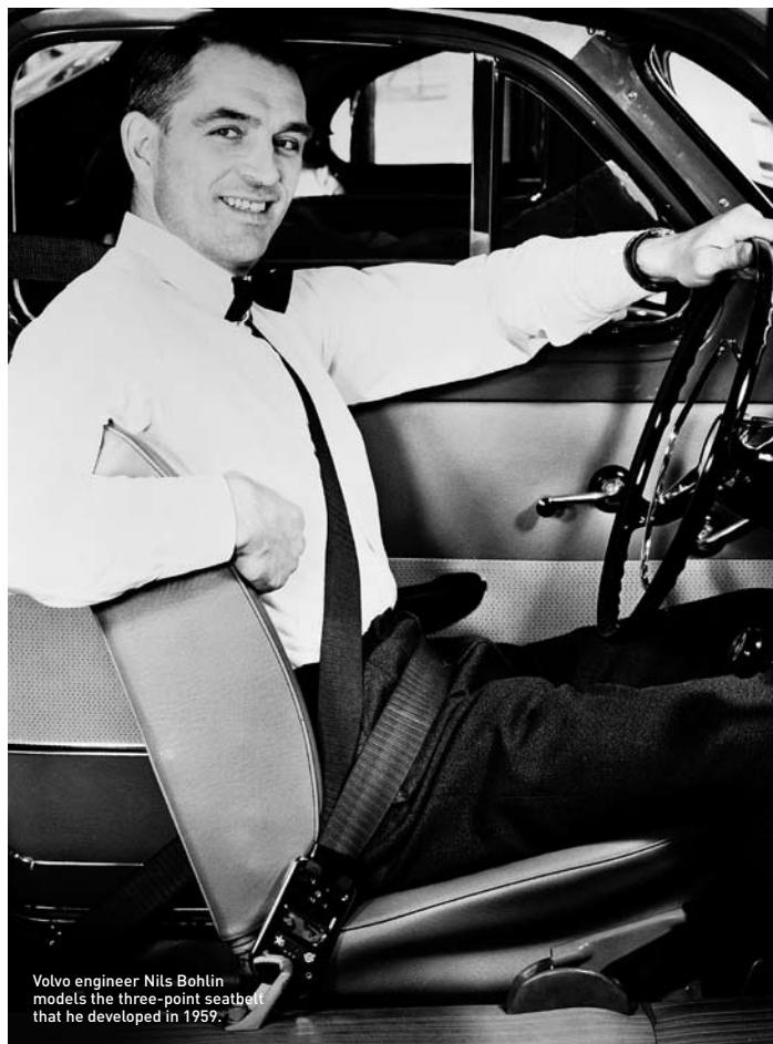
Volvo engineer Nils Bohlin models the three-point seatbelt that he developed in 1959.
